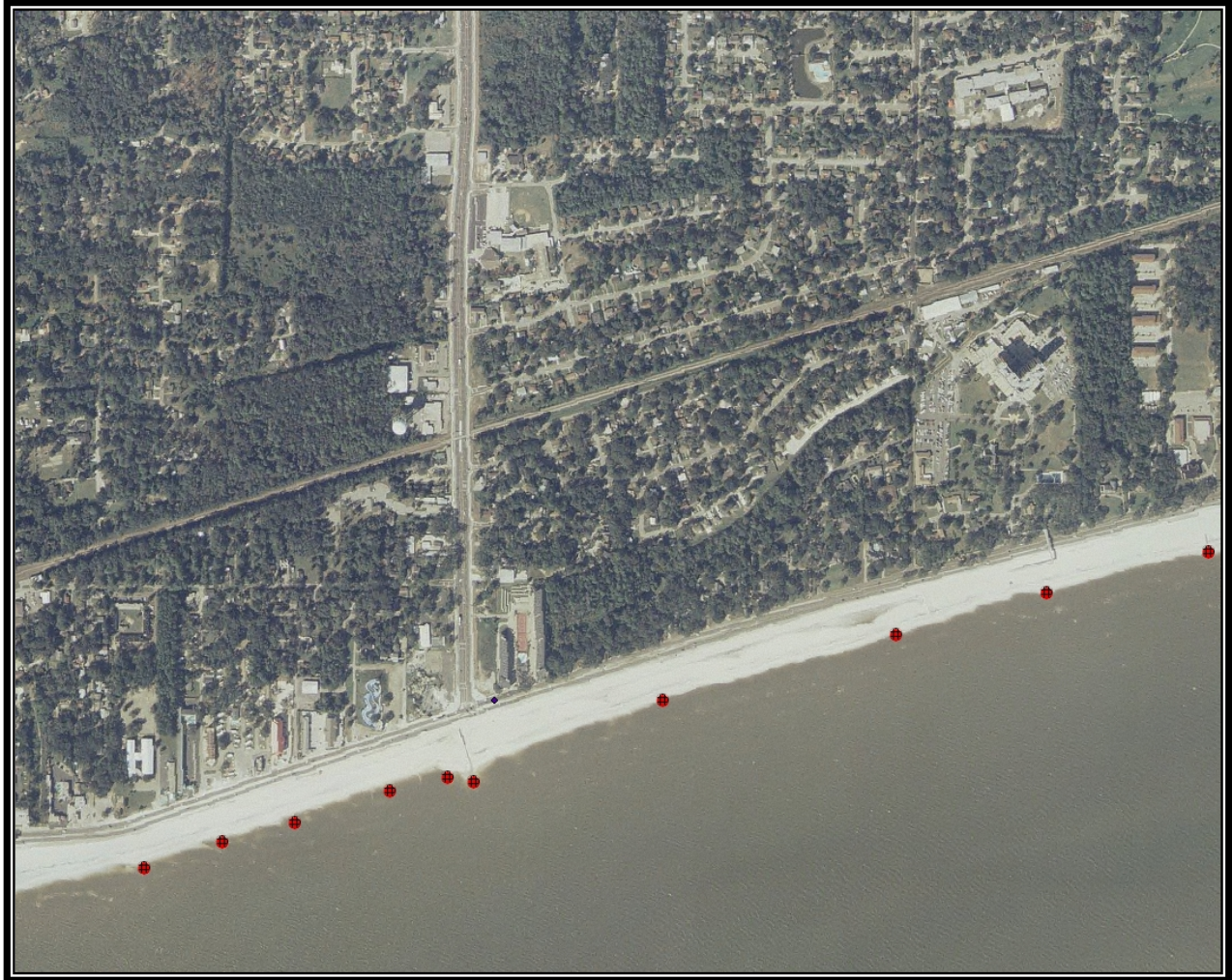
Culverts shown by red circle, lift station shown in black diamond
