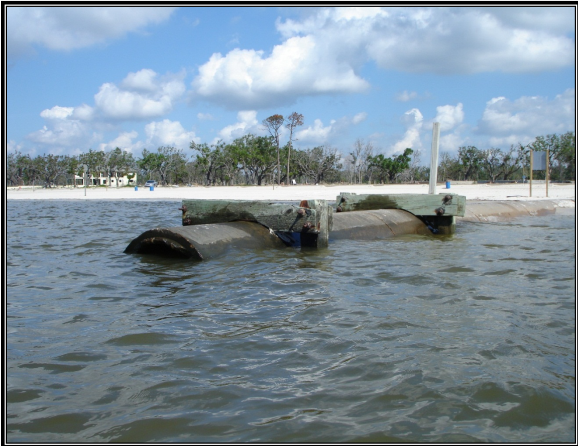
Typical Storm Water Culvert discharging on the Beach
